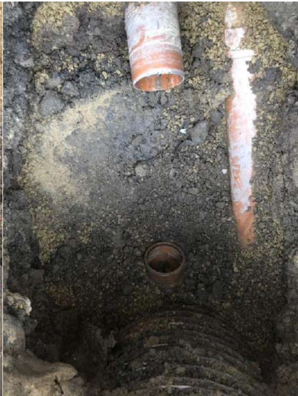
Bends removed to facilitate repair.
