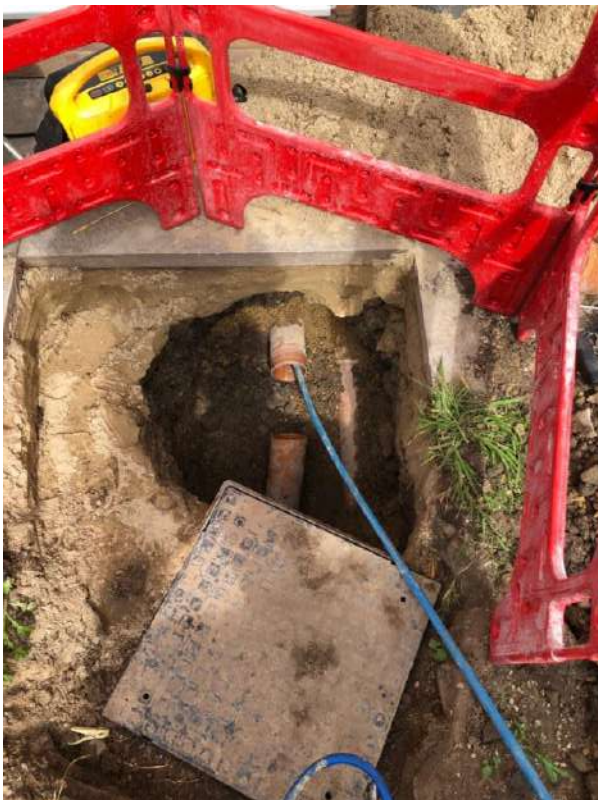
Patch repair installation from excavation.
