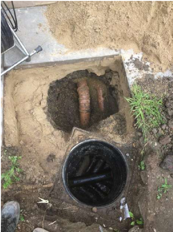
Dig down to exposed pipe with bends.
