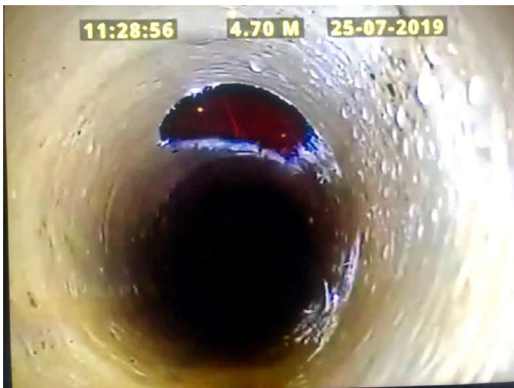
Incoming lateral covered by repair re-opened from sink.
