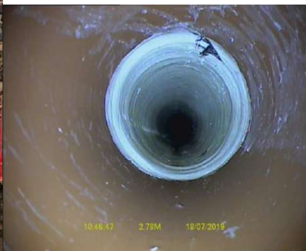
Patch repair in place.
