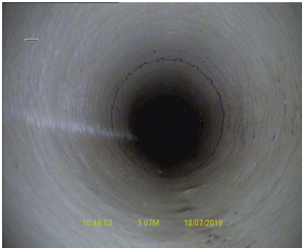
Inside the patch repair.
