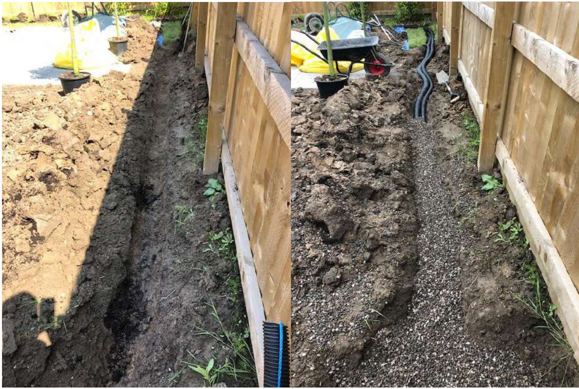
Trench dug along back fence for land drain to be installed.
