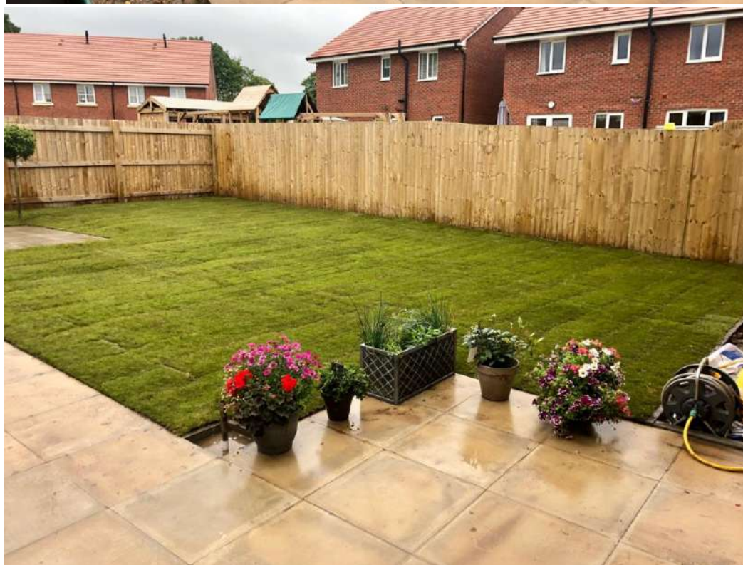
Garden upon completion of drain install and turf laying.
